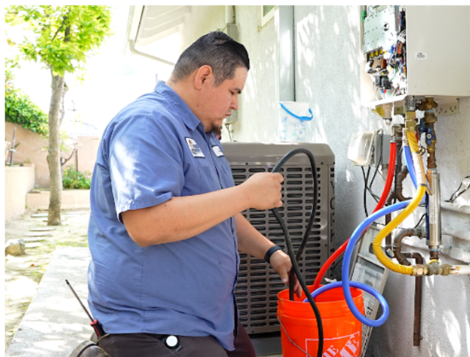
Monkey Wrench technician performing a flush on a tankless water heater.
