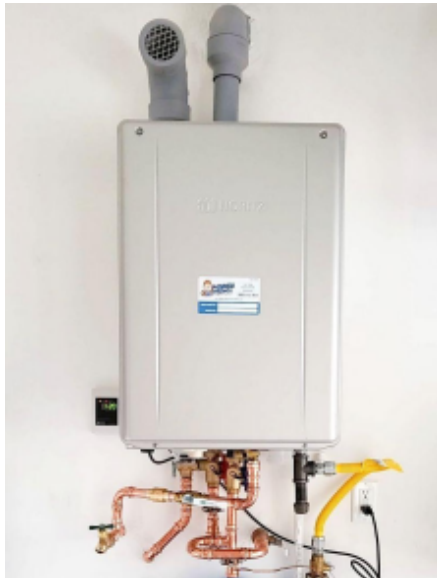
A Noritz tankless water heater mounted on a wall.
