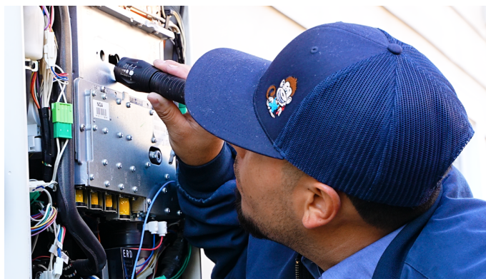
A Monkey Wrench technician inspects the inside of a Noritz tankless water heater.
